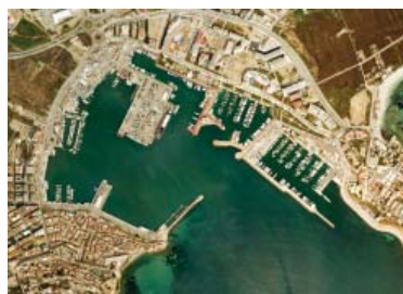
016 Porta Port Eivissa Eivissa, Spain Project 2008 Realization 2009
