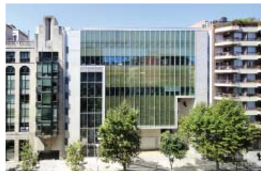
007 Edifici Collage Barcelona, Spain Competition 2007 Project 2008 Realization 2009 - 2011
