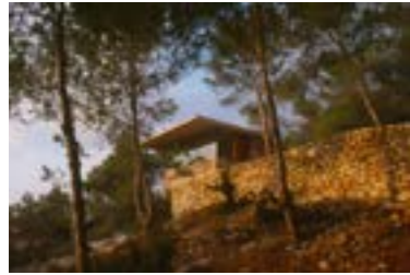
126 Pavelló Estel.la Eivissa, Spain Project 1995
