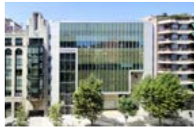
228 Edifici Collage Barcelona, Spain Competition 2007 Project 2008 Realization 2009 - 2011
