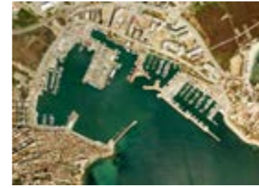
232 Porta Port Eivissa Eivissa, Spain Project 2008 Realization 2009
